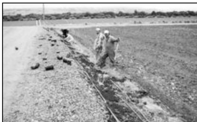
Installing short plants on a berm.
