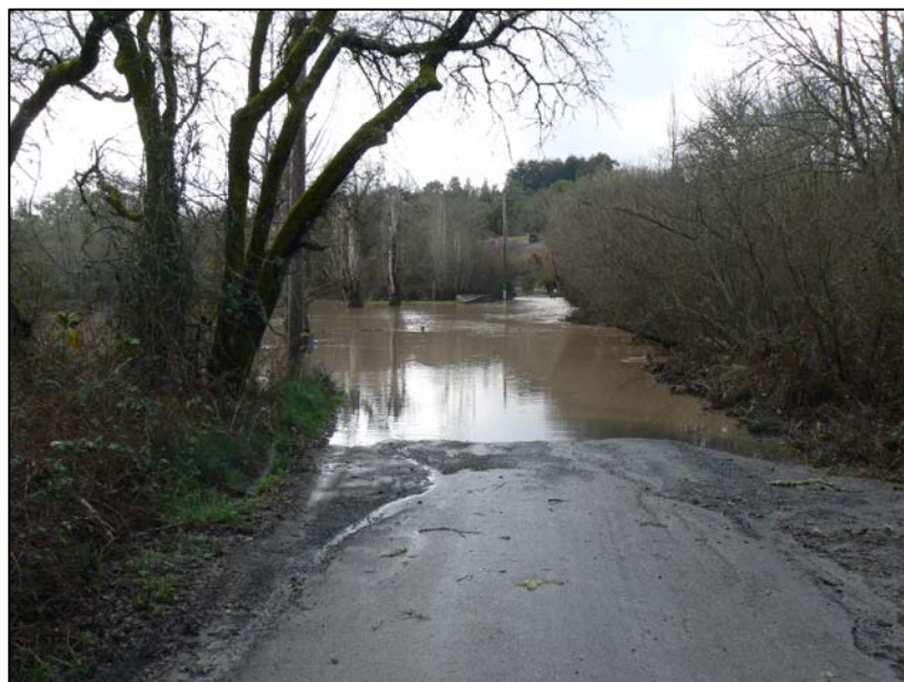
Flood flows at Ross Station Road, March 2011
