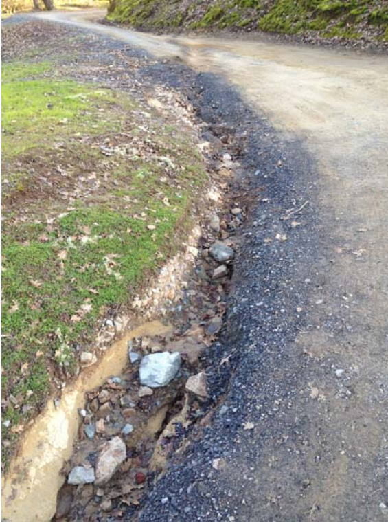
Inboard ditch. Photo courtesy of Matt O'Connor.
