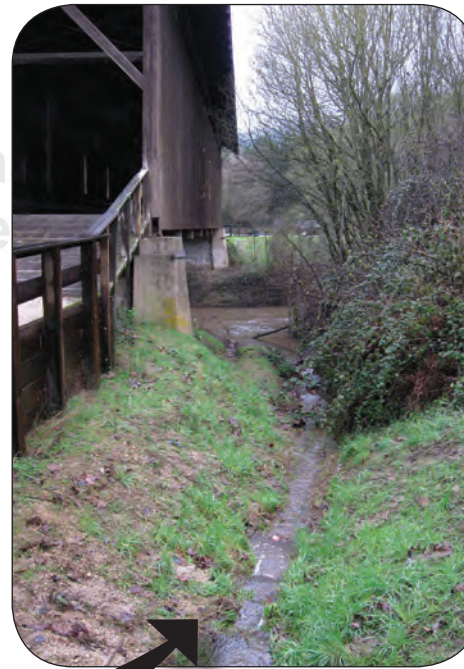
...AND CONTINUES DIRECTLY INTO LOCAL CREEKS AND RIVERS.
