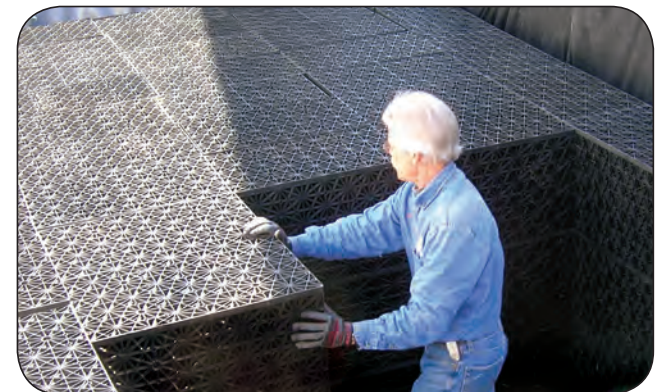
Underground systems can be customized to fit various shapes and sizes using these modular RainBoxes.
