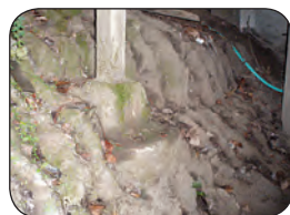
Visible erosion under a deck is common.
