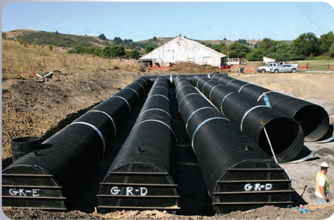
Underground rainwater storage installed at west county dairy
