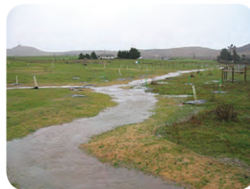
Gully repair, native plant revegetation, and exclusionary fencing
