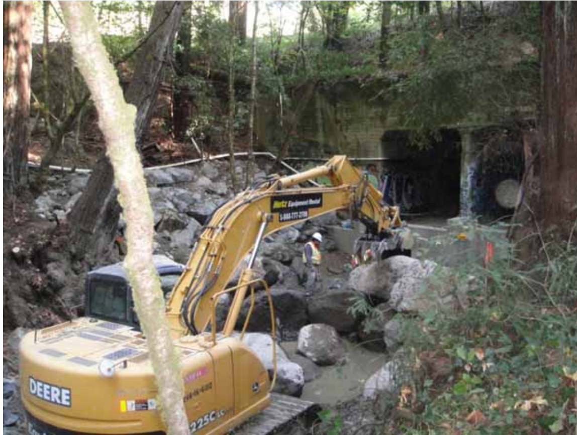
Photo # 2 of rock weir below the Market St. Culvert
