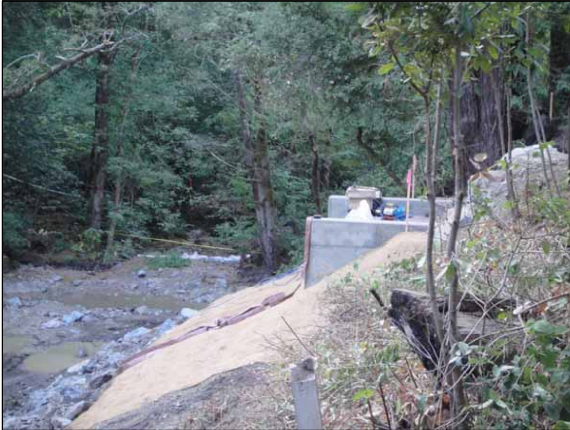
Looking downstream at foundation of bridge on the right bank
