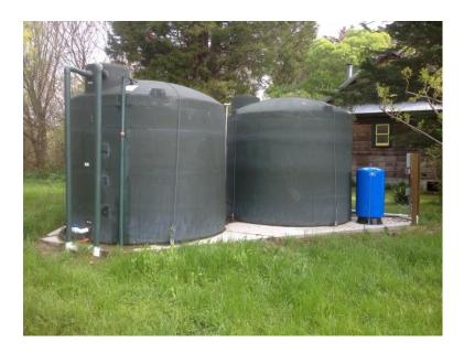
A 15,000-gallon rural residential rainwater catchment system installed through Phase I (DFW P1130404), offsetting summer diversions from a near-channel shallow alluvial well.
